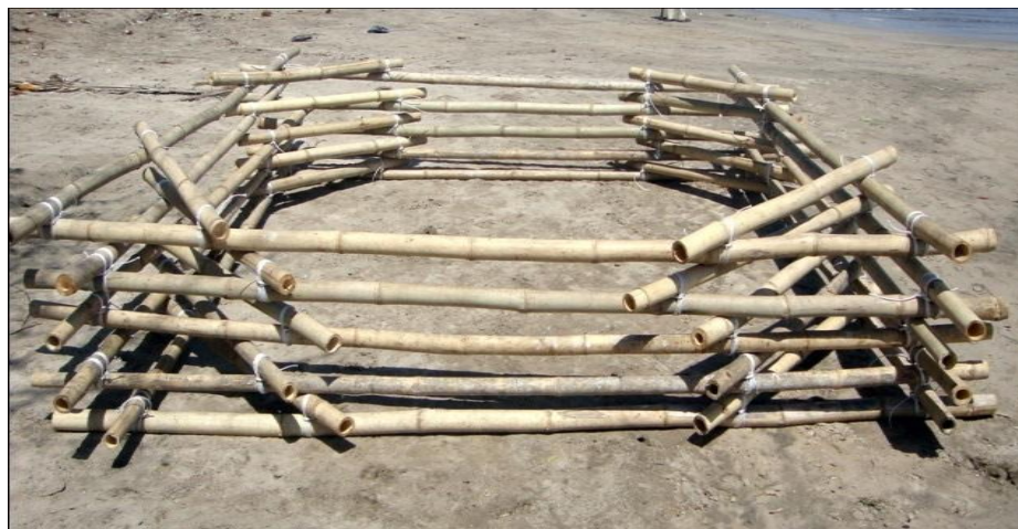
Fig : 8 Pile of fabricated bamboo rafts
