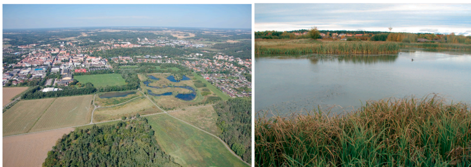
Fig. 4. Overview of Vattenparken – FWS CWs treating stormwater from Enköping (a view prior planting with macrophytes) (left), and current CW which mimics a natural habitat, providing a wide range of ecosystem services (right). Photo: Pereric Öberg (left); Tomasz Bergier (right).
