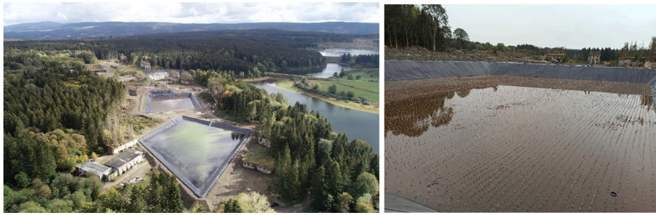
Fig. 3. Retention basin (left figure, at the bottom,), Constructed Wetland (left figure, center); Constructed wetland planted with Common reed ( Phragmites australis ) (right figure). Photo: Halali Verwaltungs GmbH, Landkreis Goslar.
