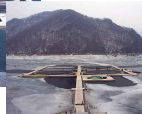
This six-tank facility in China operates summer and winter in a freshwater reservoir. During cold periods, warm water from deep below the tanks is pumped through the tanks so no freezing occurs, and fish growth continues.
