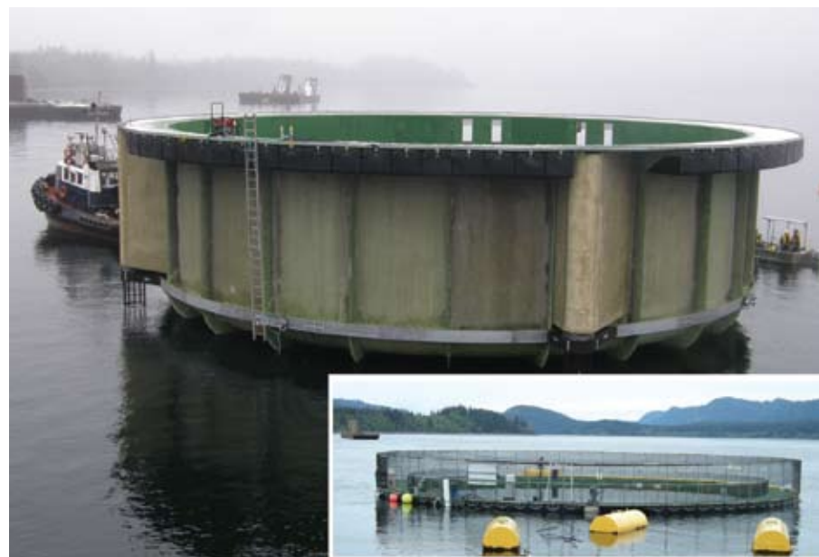
Solid-wall tanks are towed into position and “sunk” to a defined level. Safety and bird protection fence and netting are often added.
